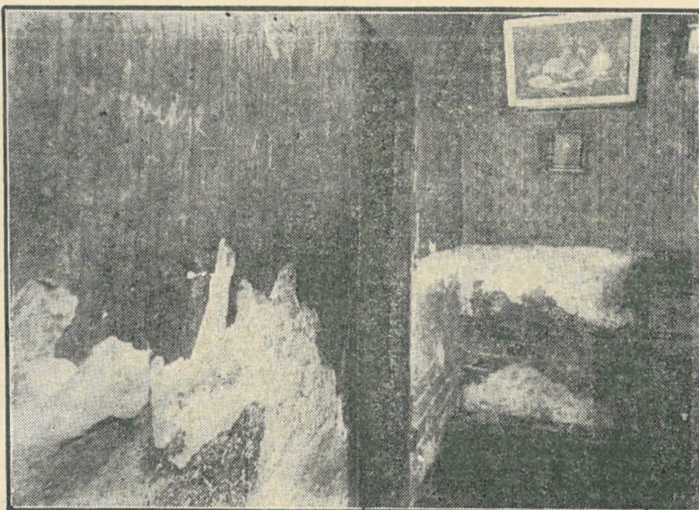
A view of the walls of the living room of another house in the same court. It will be seen that not only is the paper off the wall, but also the plaster, exposing the bricks and mortar beneath.
